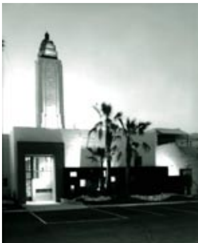
View of rear entry
